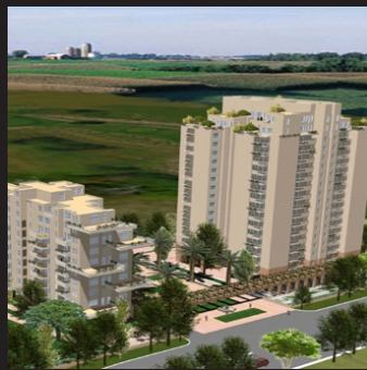
Aloha Housing Gurgaon
